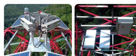
Thanks to its in-house design office, DELTA BOX can design customized solar power station to supply power to AWL systems installed in remote areas. The dimensioning takes into account the AWL system consumption, as well as the solar insulation of the geographic area where the system will be installed. Batteries capacity is calculated to optimize the lifetime.
